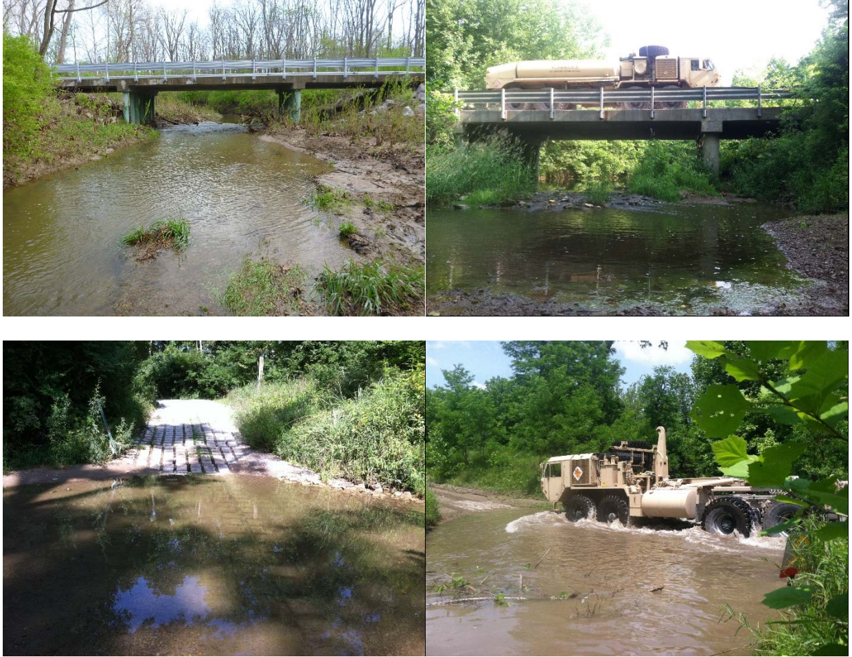
Figure 3.2. Nineveh Creek crossings CA1-CA4 (starting at upper left and going clockwise)
