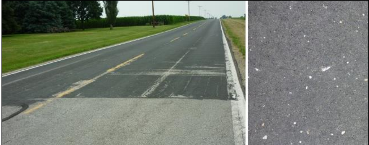
Figure 5.30: Second 1-mile Segment of County Highway 32 (newly placed surface treatment)
