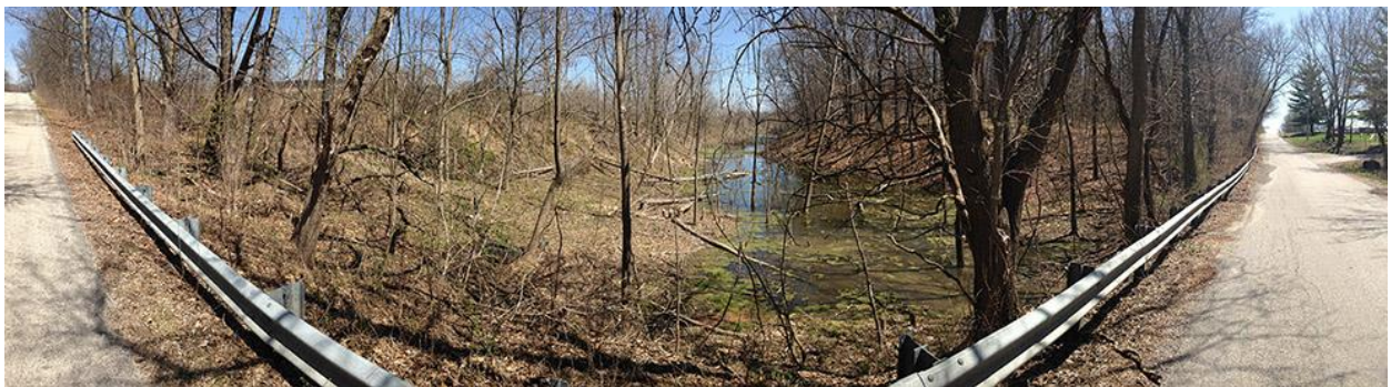
Figure 2.2: Looking east across an open tributary leading to the Vermilion River along the southern edge of the Brickyard active landfill. Trash, algal blooms and intense odor present during several observations.
