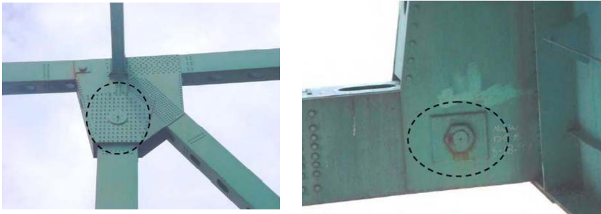
Figure 4.43 Truss intermediate hinges
