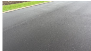
Church St (Sections 3 and 4) after Overlay
