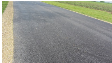
East Coral Road (Sections 1 and 2) after Overlay
