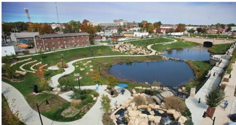
Figure H.4: Regional detention basin in Champaign, IL. Photo courtesy of FOTH.
