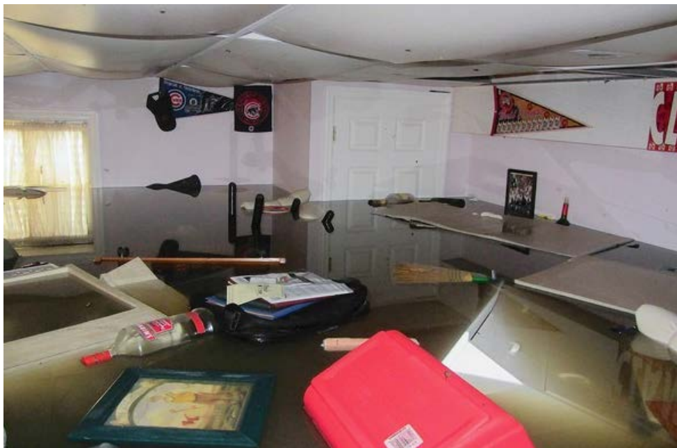
Figure C.2: Lake Zurich basement, June 2013 (Chicago Tribune, Dan Waters)
