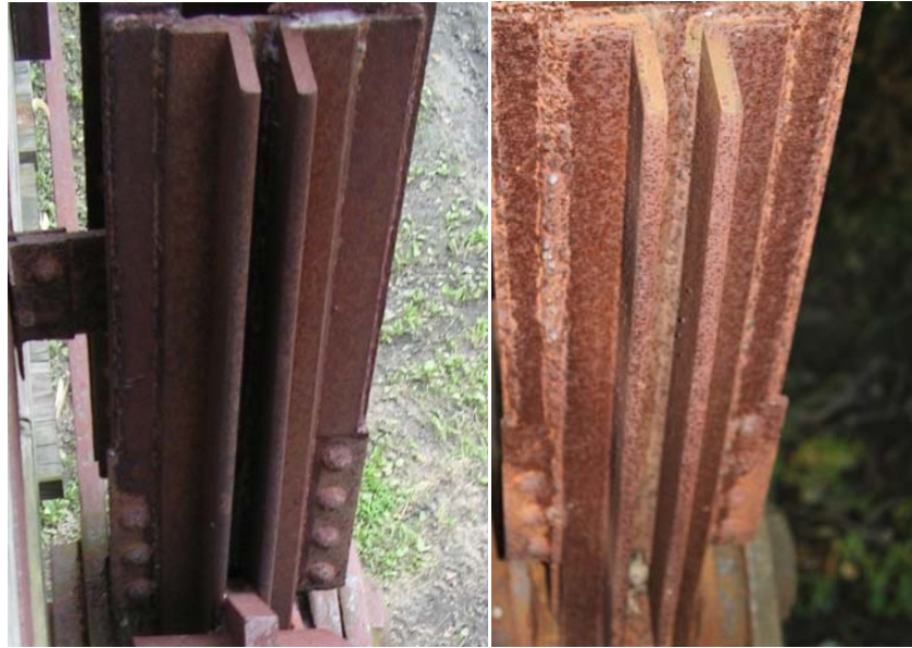
Figure 8.29. Retrofitted plates in 2008 (left) and in 2010 (right).
