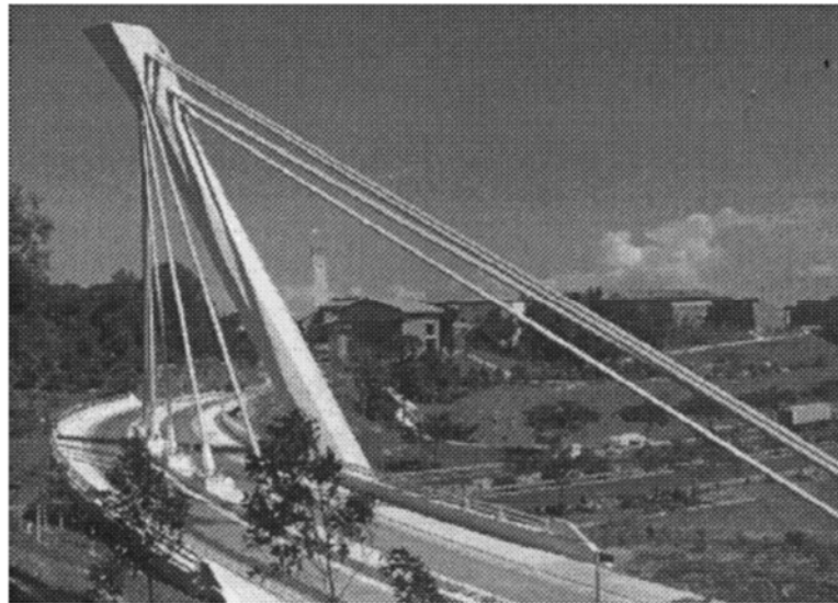
Figure 2.3. Safti Link Bridge (Courtesy of Brownjohn, 2000).
