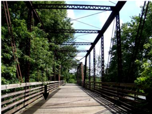
(a) Timber deck
