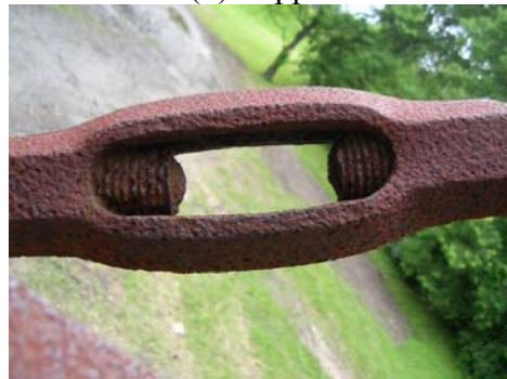
(c) Connections: rivet and bolts
