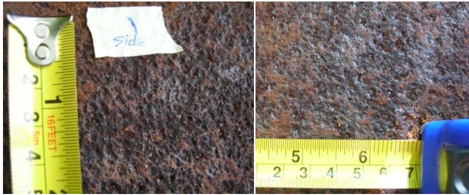
(a) Section 1 in 2008 (left) and in 2010 (right)
