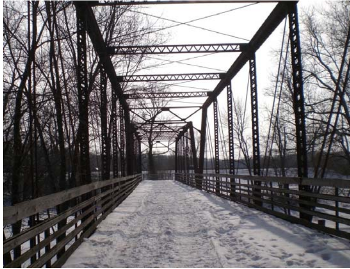
(a) Mahomet bridge on January 14, 2010
