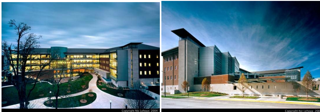
(a) North exterior
