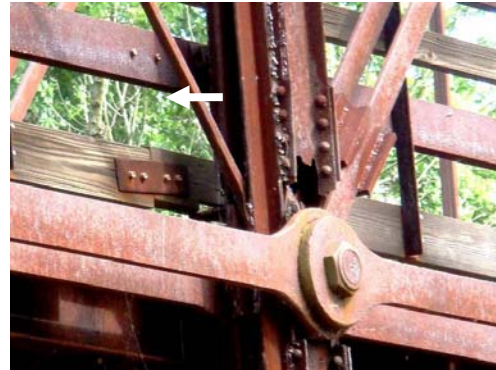
(b) Retrofitted vertical chord
