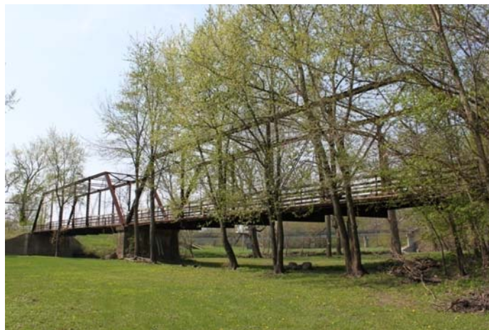
Figure 7.1. Mahomet Bridge, Illinois.
