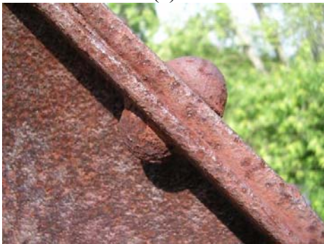
(c) Connections: rivet and bolts
