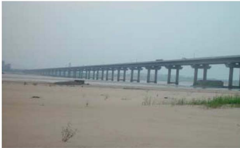
Figure 2.4. Photograph of Hongtang Bridge (Courtesy of Jaishi, 2007).
