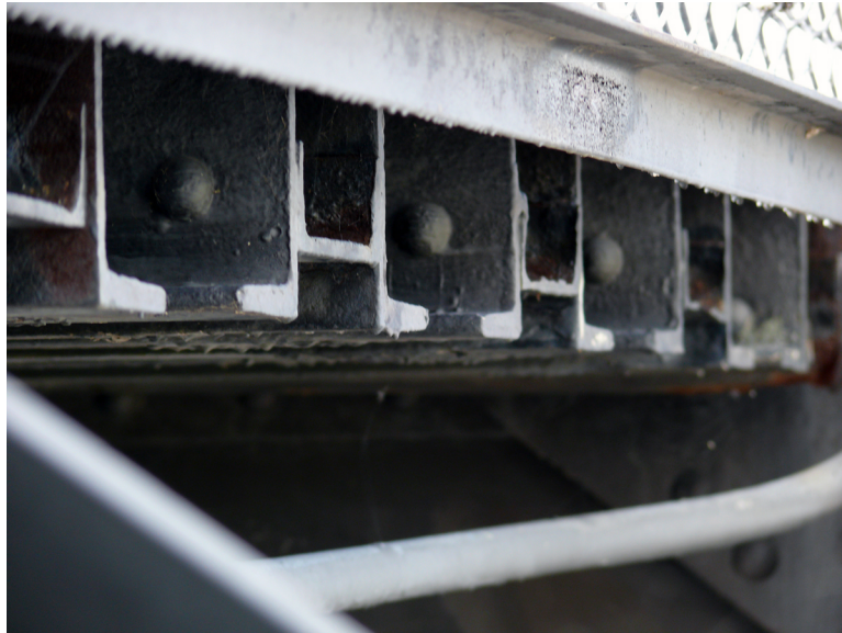
Figure 6.6: Close up view of the built-up corrugated railroad deck.
