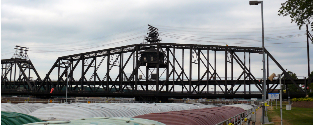
Figure 1.2: Span II (swing span) with barges entering lock.
