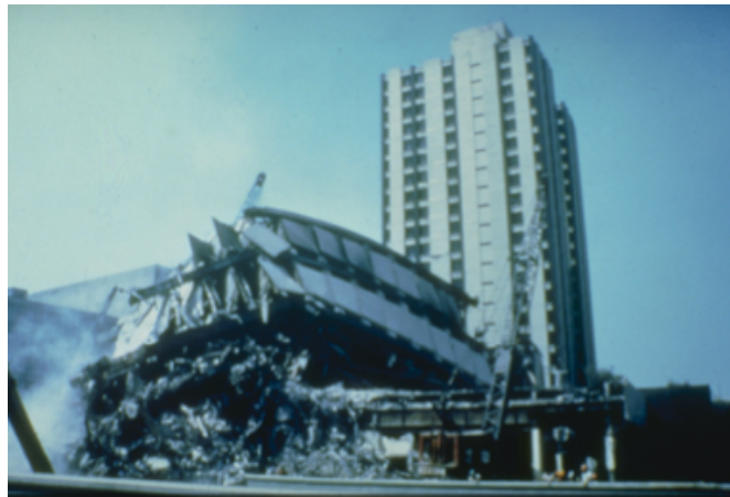
Figure 2.3 Wreckage of a 22- story steel-constructed building in the Pina Suarez Apartment Complex in 1985 Mexico City earthquake comparing to the identical building standing in background (Photo credit: National Geophysical Data Center, NOAA, E.V. Leyendecker, National Bureau of Standard).
