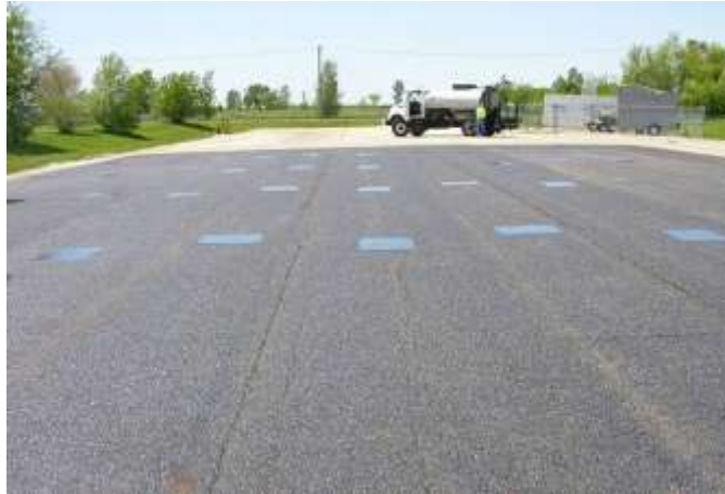
Figure 3.13 Existing pavement surface after tack coat application.
