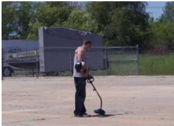
(a) Surface cleaning with an air blower.
