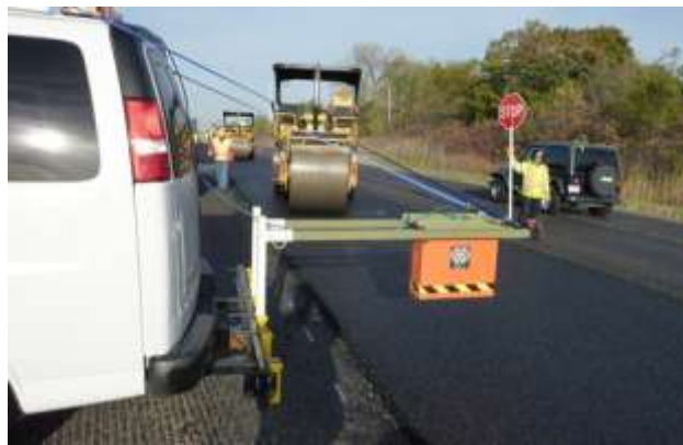
Figure 3.34 GPR data collection during compaction.
