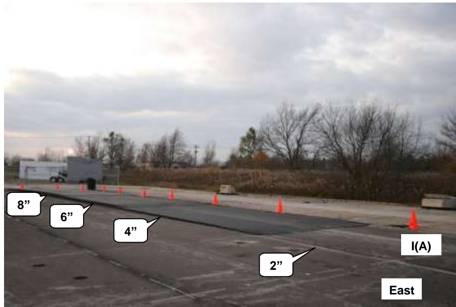
Figure 3.21 Lane I(A) after the second-day construction.
