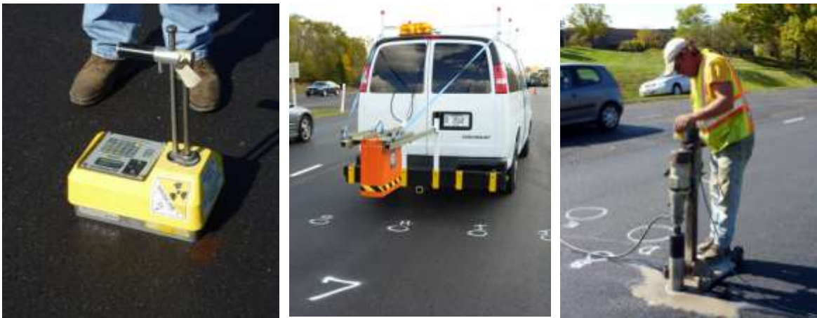
Figure 3.35 In-service pavement data collection: (a) nuclear gauge testing; (b) GPR data collection; (c) core extraction.
