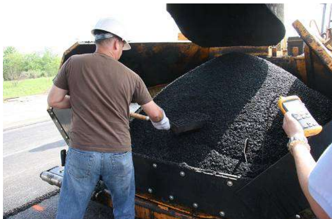
Figure 3.16 Sample collection from the paver.
