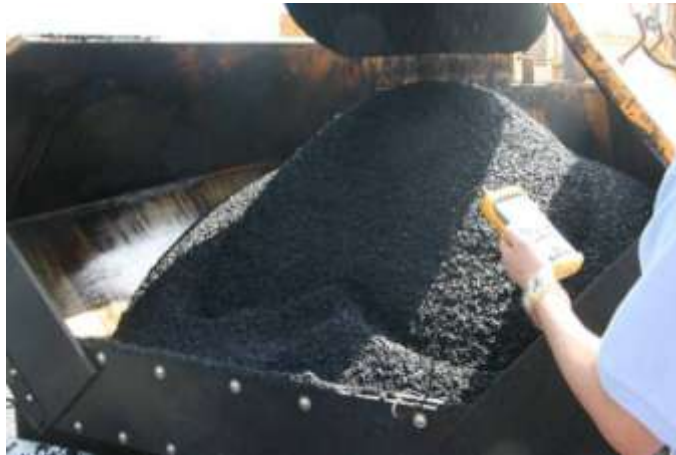
Figure 3.17 Mix temperature check using a temperature probe.
