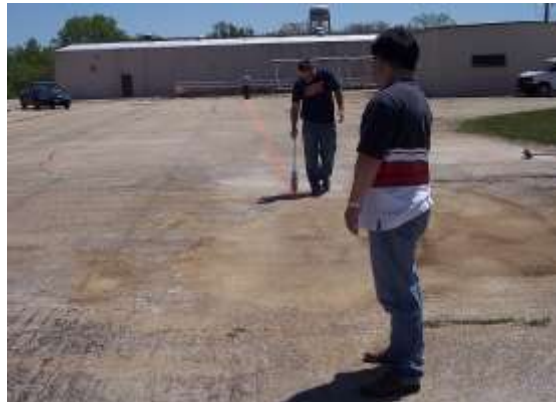
(b) Surface marking using paint.
