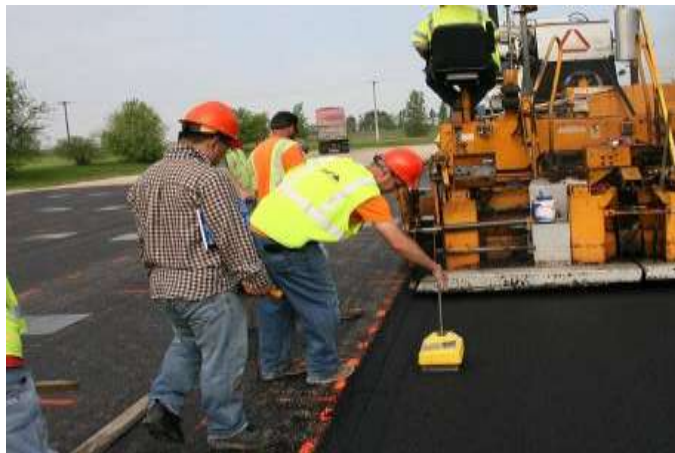
Figure 3.19 Density measurement using a nuclear gauge.
