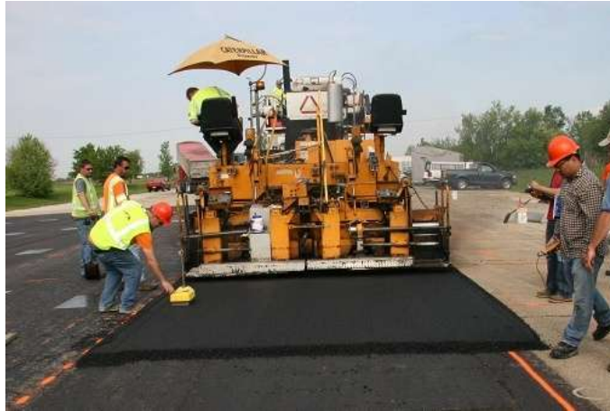
Figure 3.14 Paving the first lane.
