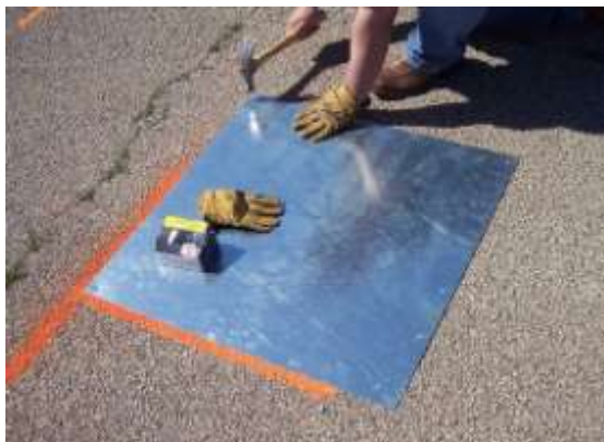
(c) Fixing the steel plate using nails.
