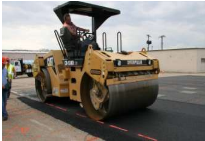
Figure 3.18 Pavement compaction.
