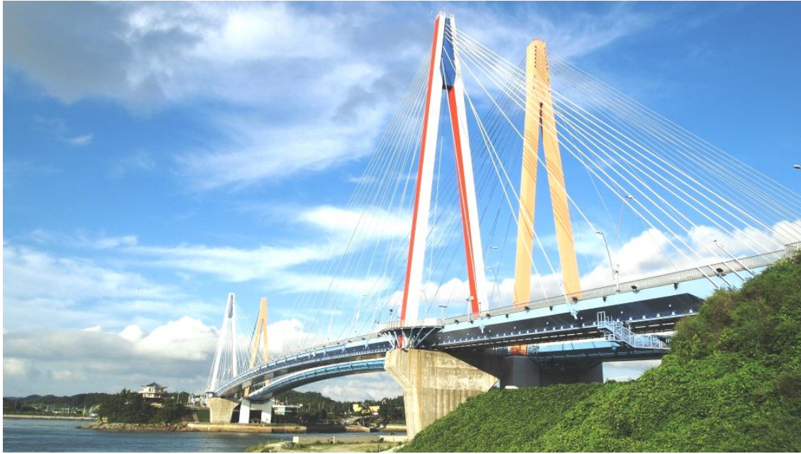
Figure 7.1. The Jindo Bridges.
