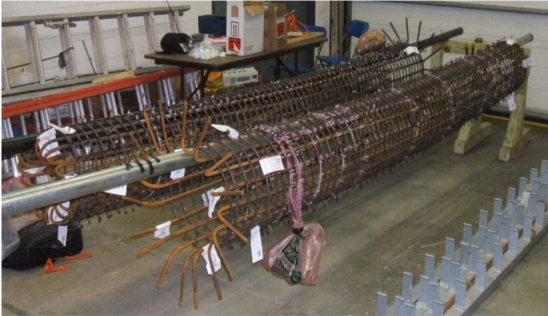
Figure A.5 Reinforcement cages of 1:3 scale piers
