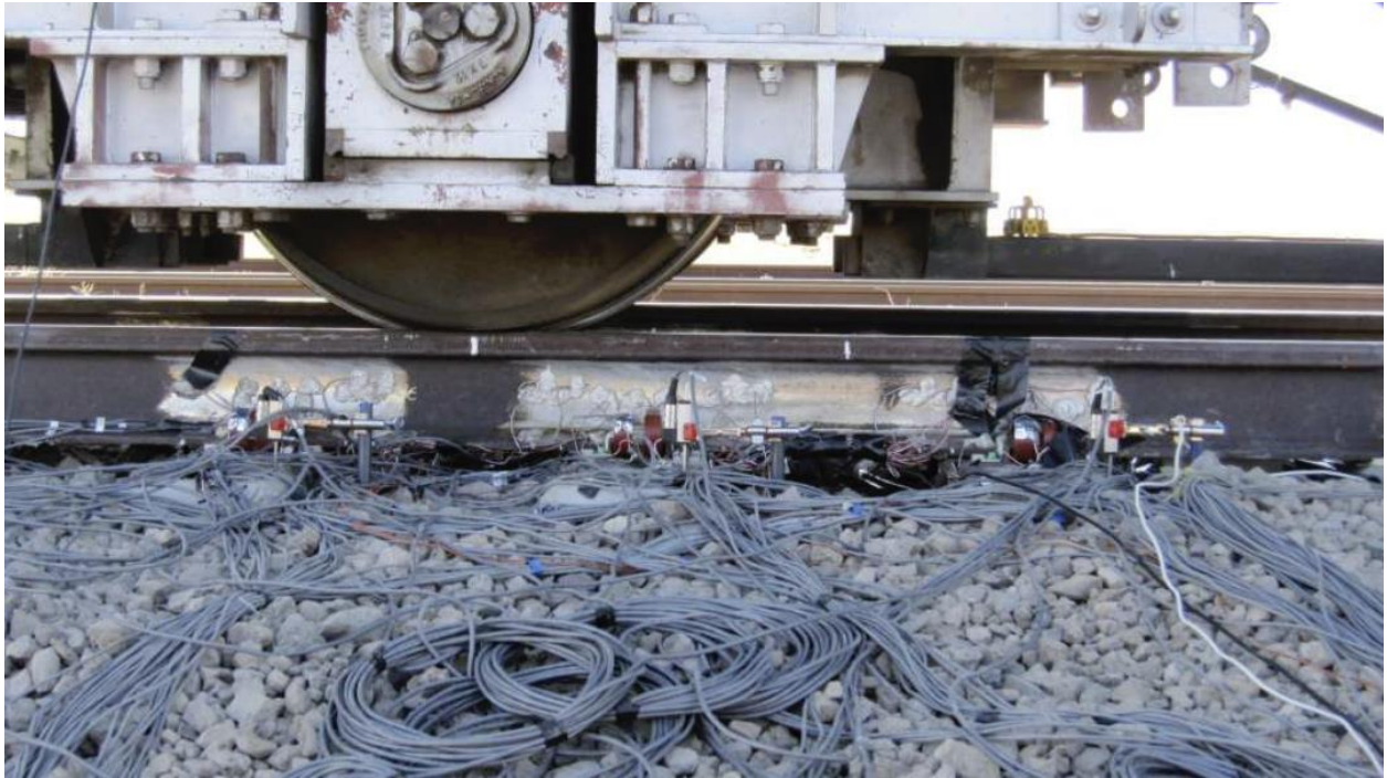
Figure E7: TLV applying load between fully instrumented rail seats.
