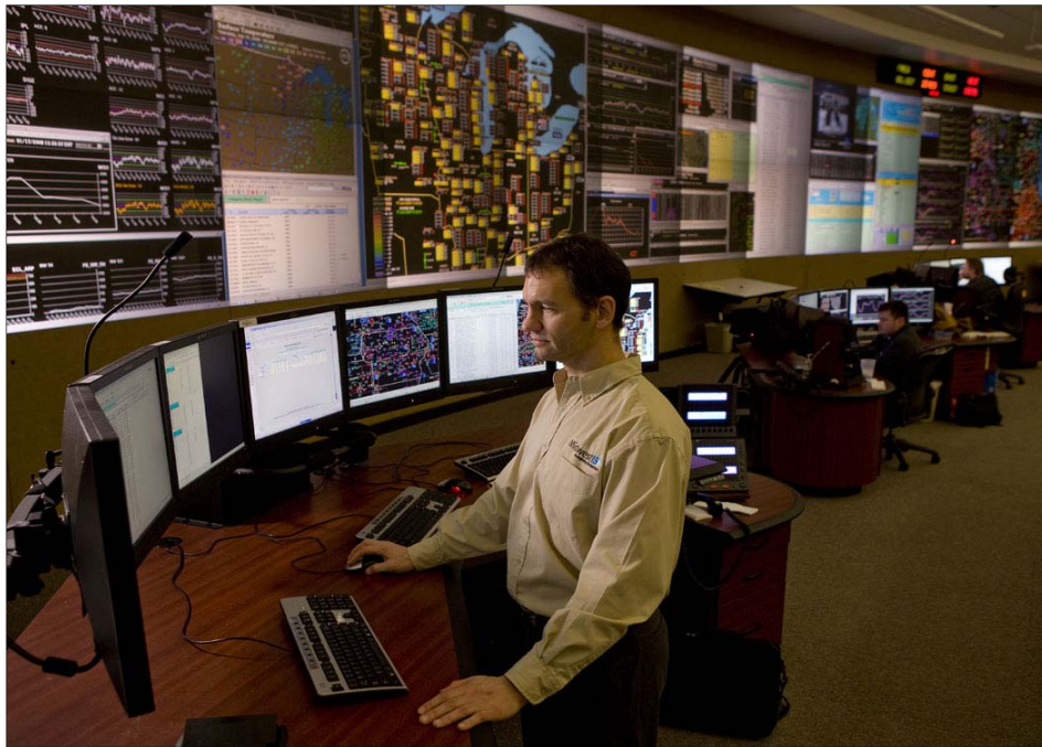
Figure 12: MISO control center in September 2009 (Source: MISO)
