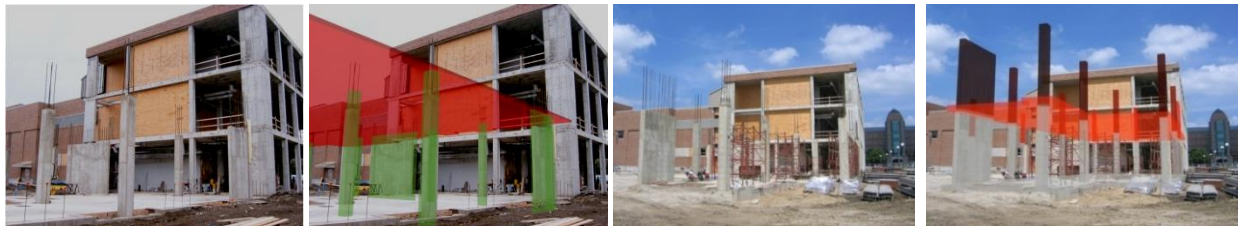
Figure 28. Randomly taken photograph of the construction site and the superimposed photograph representing progress status: From Left to Right: First two photographs: 11-07-06, 10:00AM, Second Two photographs, 11-08-2007, 11:20AM, UIUC College of Business Instructional Facility.
