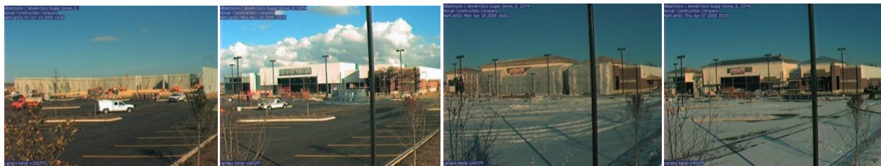
Figure 33. Time-lapsed photographs taken during construction of Jewel Osco, Sugar Grove, IL
