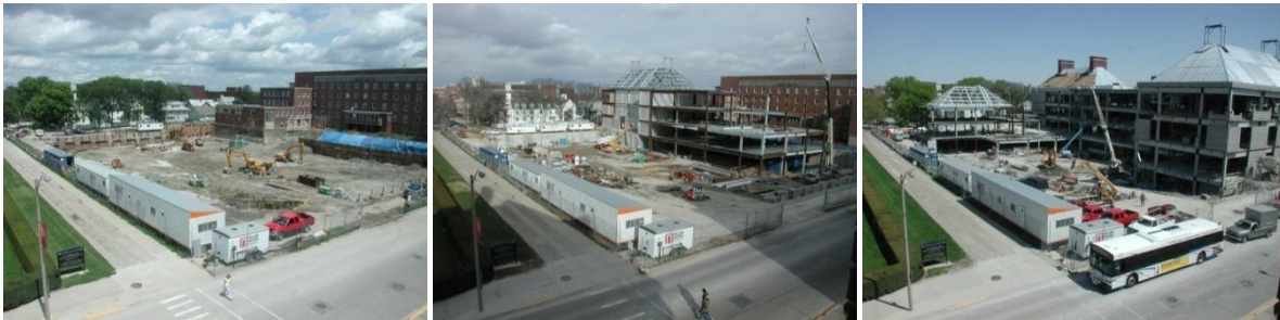
Figure 30. Photographs taken during construction of Institute of Genomics Biology, Champaign, IL.
