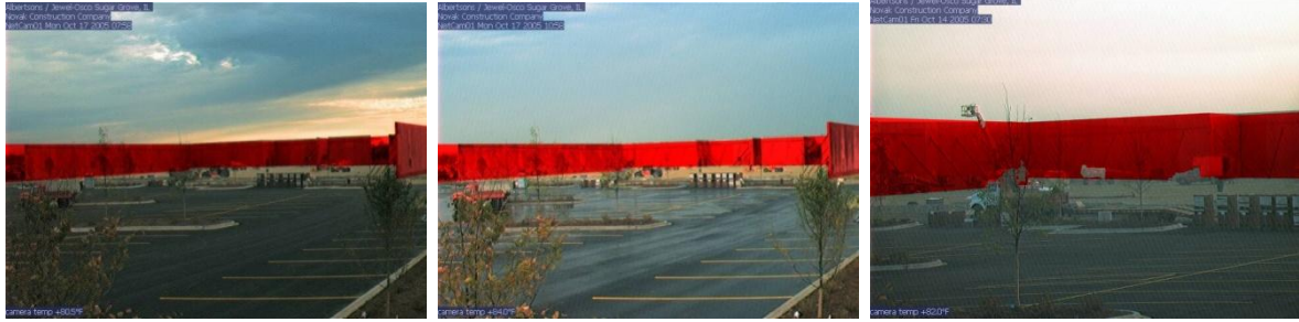
Figure 34. Snapshot of the Jewel Osco 4D model and a superimposed photograph visualizing the progress status, Jewel Osco, Sugar Grove, IL.
