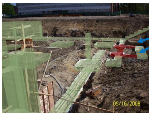
Figure 3.16. The superimposed photo visualizing the component which has been misinterpreted by the carpenter foreman. Student Dining and Residence Hall project, Champaign, IL. Photograph courtesy of Turner Construction Company; Champaign, IL; used by permission.
