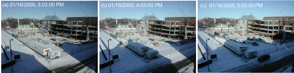
Figure 2.4. Effect of shadow on a single working day (Photograph subject: Institute of Genomics Biology, UIUC; Source: Information, Technology & Communication Services, College of ACES, UIUC).
