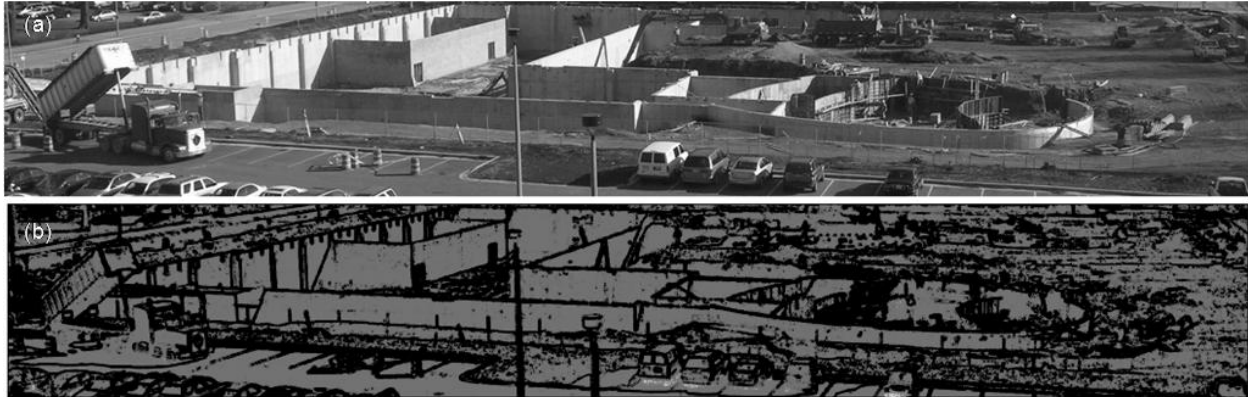
Figure 2.13. (a) Cropped portion of the photograph taken on 01/03/2007; 11:22:55AM and (b) the image after applying SUSAN Edge detection algorithm (Threshold=20); as seen the excavation line, lamp posts, truck on the left side of the photograph and the cars parked are recovered.
