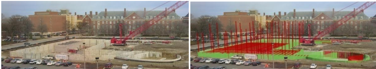
Figure 20. Time-lapsed photograph of the construction site and the superimposed photograph representing progress status, 01-08-2007, 11:10AM, UIUC College of Business Instructional Facility.
