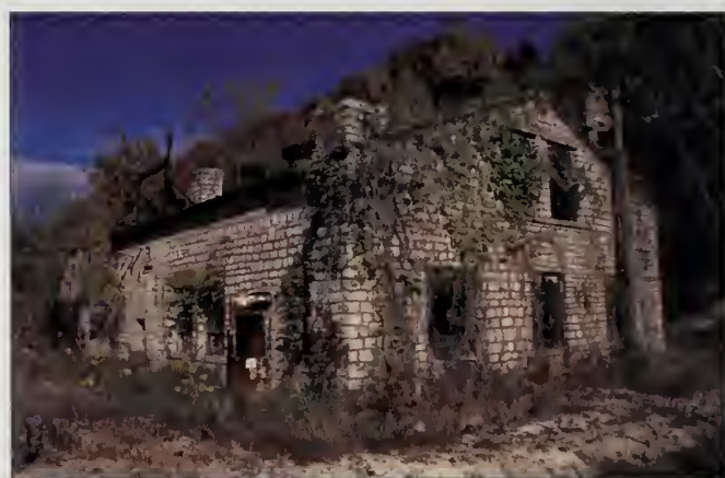
Figure 31 This now abandoned building at Valmeyer Quarry is another example of the use of natural materials for construction in southwestern Illinois (Panno et al. 1999).
