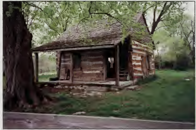
Figure 21 This two-story log cabin was built by the Stemlers in 1836 and overlooks a large sinkhole just to the south that is the entrance to Stemler Cave. The property was chosen by the Stemlers in order to use the cave for storage of eggs and dairy products during summer months (Homer Stemler, personal communication 1995). (Photograph by Samuel V. Panno.)
