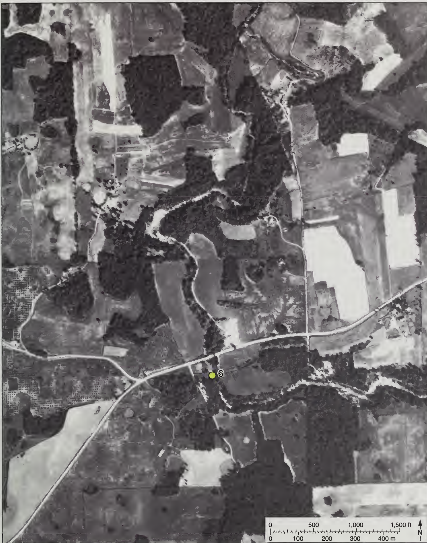
Figure A12 USDA-AAA aerial photograph of the Fountain Creek Stone Bridge area and associated karst terrain acquired on September 5, 1940.
