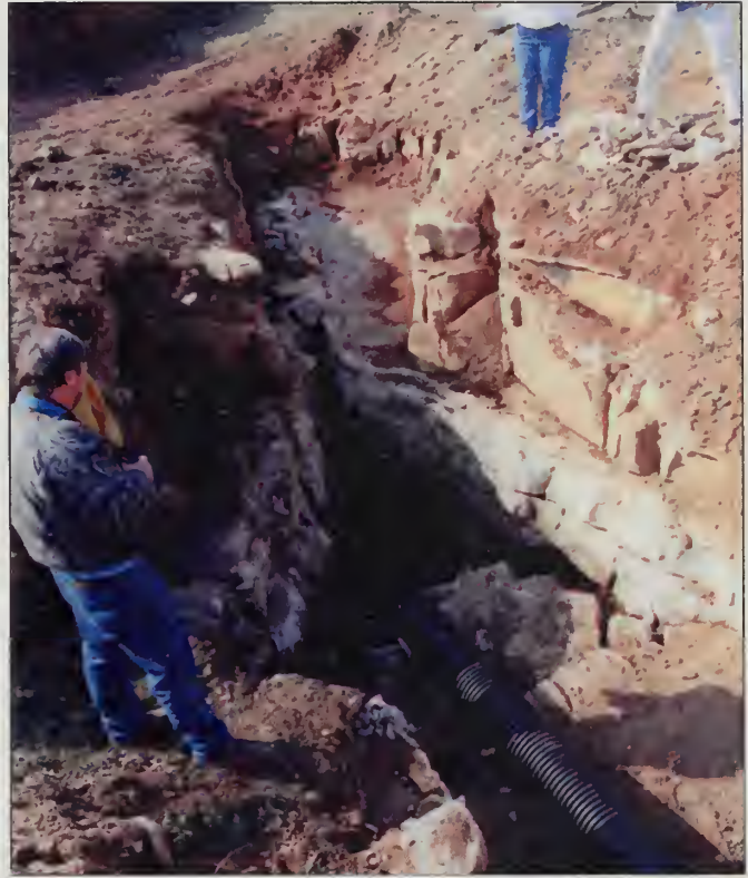
Figure 4 The excavation of a 100-m diameter sinkhole revealed a narrow crevice in the exposed St. Louis Limestone bedrock that leads to a somewhat wider crevice. The wider crevice led down, about 5 m, into a small cave about 0.3 m high and 0.6 m wide through which runoff from rainwater and snowmelt flows (Panno et al. 2009).
