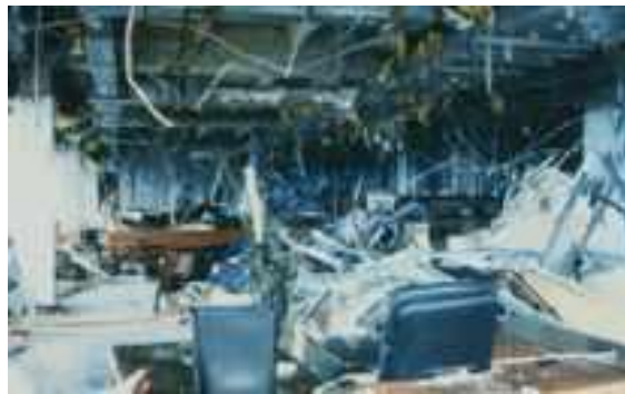
Figure 3. Burger King Headquarters' CEO office in Miami after Hurricane Andrew (NHC, 2010)
