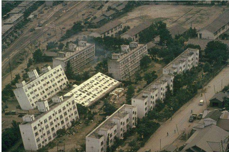
Figure 9. Collapse due to Liquefaction (Isaradharm, 1997)
