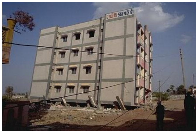
(c) 2001 Gujarat Earthquake (SED, 2011)
