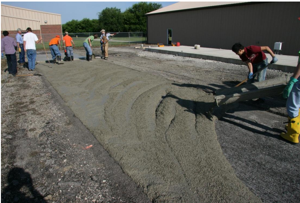
Figure 2-12 Photograph from construction of the FFC inlay.
