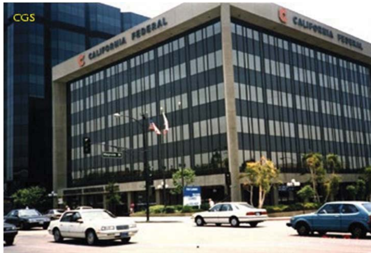
Figure 6-1 Photo of 6-story steel moment frame building in Burbank, California
