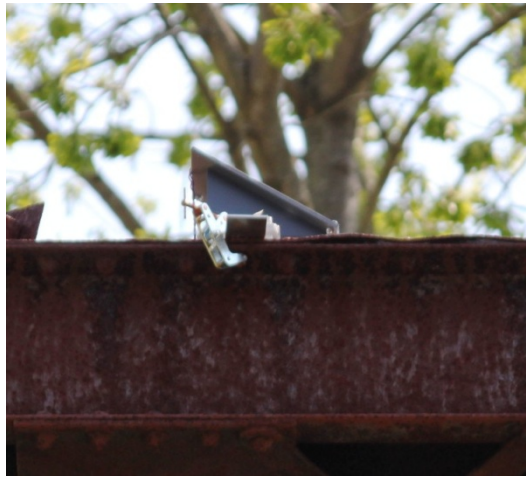
Figure 8.11. Sensor on the upper chords.
