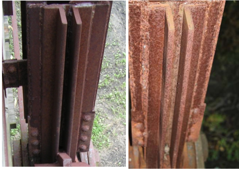
Figure 8.30. Retrofitted plates in 2008 (left) and in 2010 (right).
