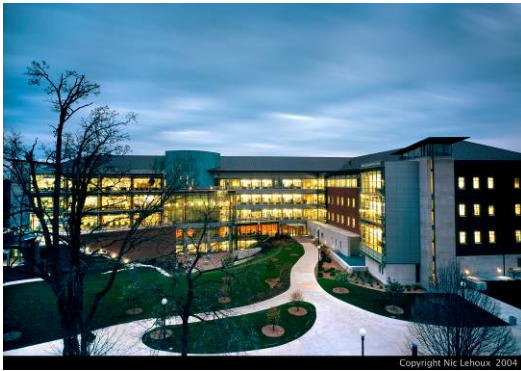
(a) North exterior
