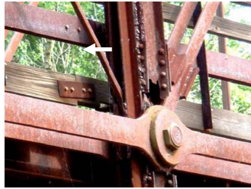
(b) Retrofitted vertical chord
