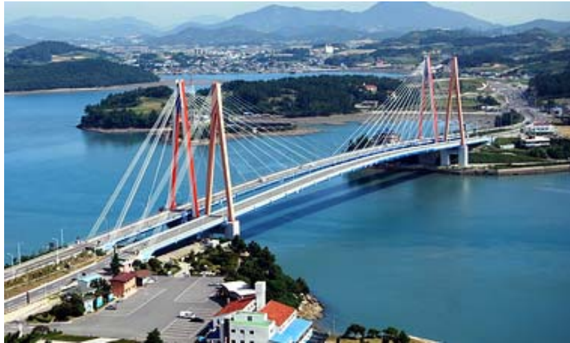
Figure 6.1. 1 st (right) and 2 nd (left) Jindo Bridges.
