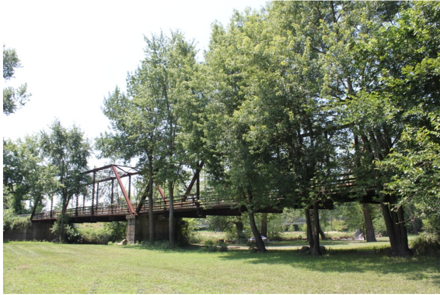
(b) Mahomet Bridge on July 2, 2010
