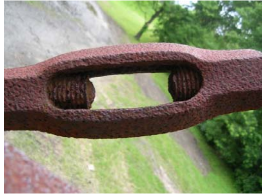
(c) Connections: rivet and bolts
