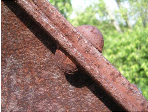
(c) Connections: rivet and bolts
