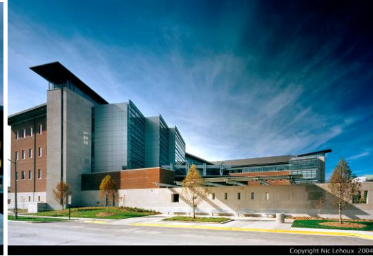
(b) South exterior
