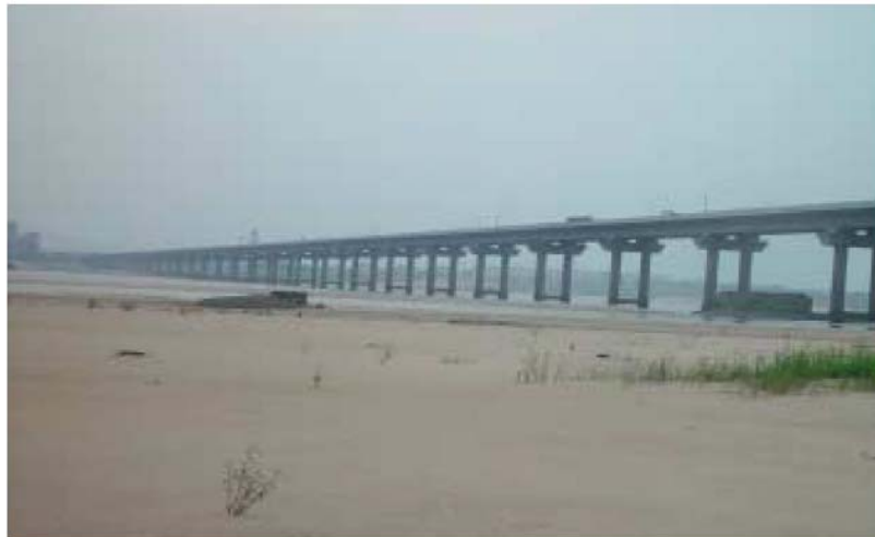
Figure 2.4. Photograph of Hongtang Bridge (Courtesy of Jaishi, 2007).
