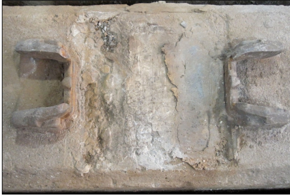
Figure 3.4 Typical example of RSD, showing wear of the steel shoulder (on the left), the top layer of cement (exposed aggregate on the left), and the polyurethane coating (still intact on the right)
