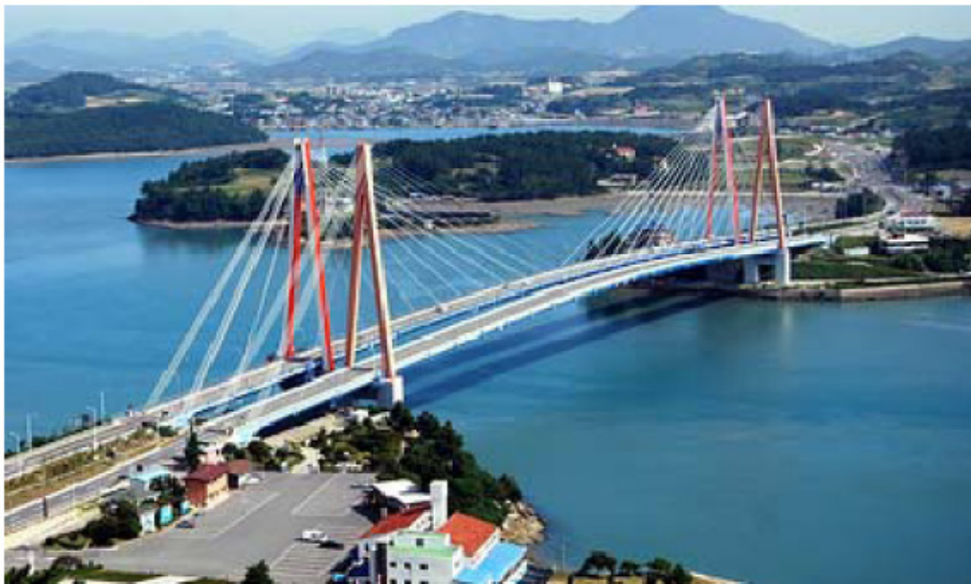
Figure 6.2 Twin spans of Jindo Bridge connecting Jindo Island with the Korean Peninsula with the newer span on the left (Rice et al, 2010; Jang et al. 2010).
