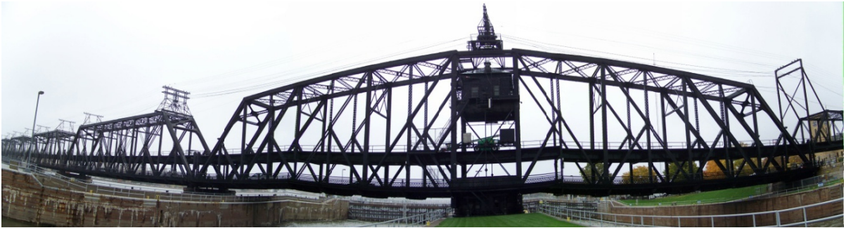
Figure 6.8 Government Bridge draw span in Rock Island, Illinois.
