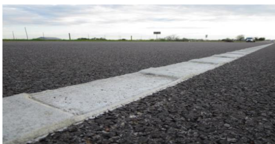
(a) Profiled Pavement Marking
