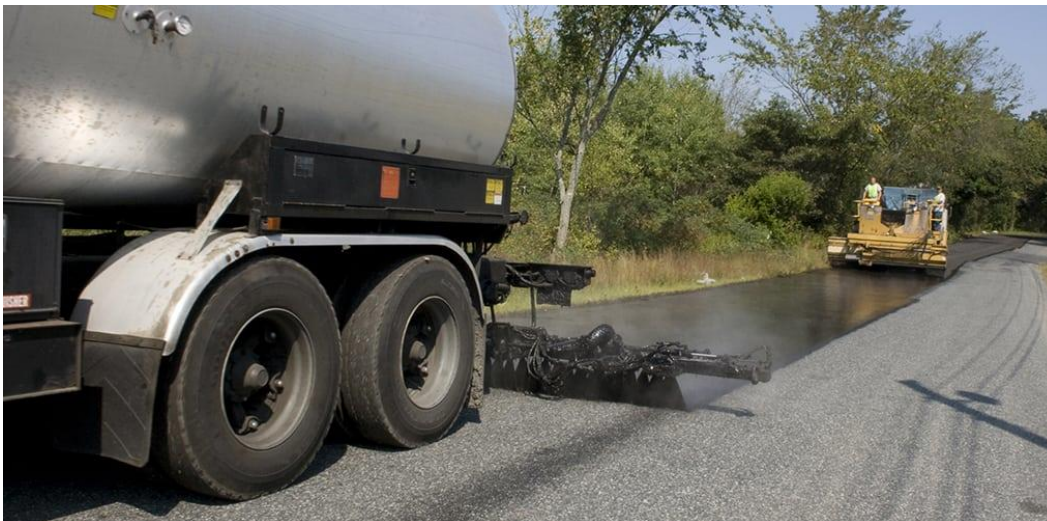
Figure 109. Photo. Chip seal application.
