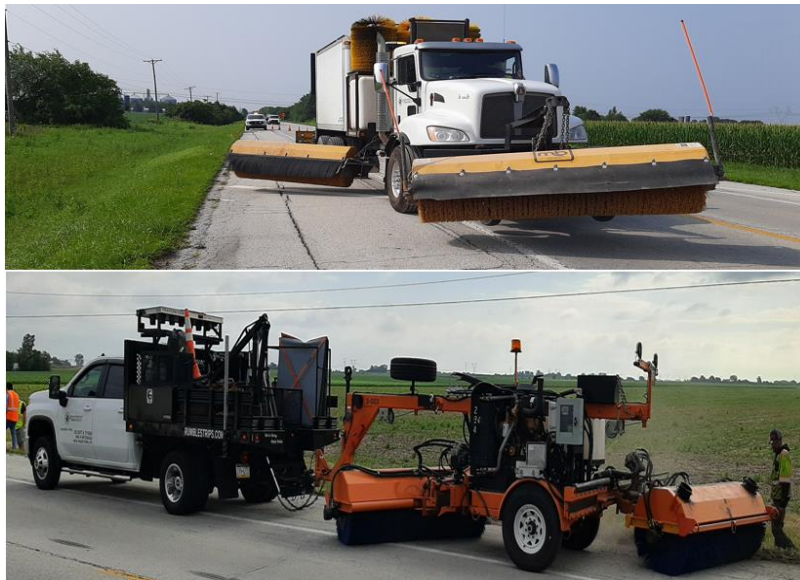
Figure 14. Photo. Roadway sweeping.
