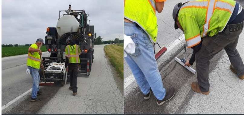
Figure 13. Photo. Rumble strip milling and quality control procedures.
