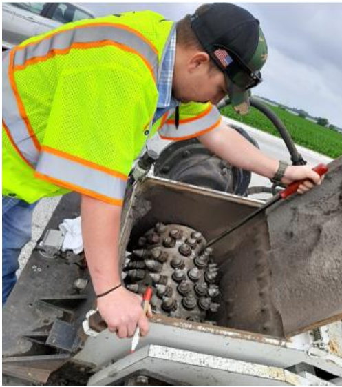
(a) Milling drum for traditional rumble strip
