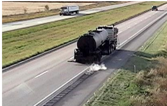
Figure 118. Photo. Fog seal application on rumble strips.
