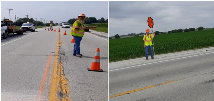
Figure 12. Photo. Lane closure and traffic control.
