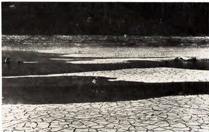
Deposited sediment takes space intended for water storage
