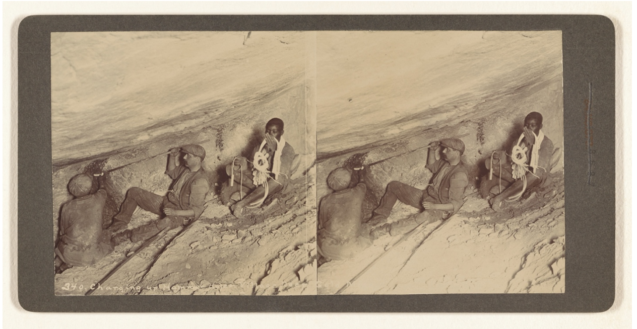
J. Wilbur Read, Charging up Hammer Holes. Village Deep (---Illeg.) (Recto); Cutting a Timber, Village Deep. (Verso) , about 1910, Gelatin Silver Print, about 1910, J. Paul Getty Museum, https://www.getty.edu/art/collection/objects/92383/j-wilbur-read-charging-up-hammer-holes-village-deep-illeg-recto-cutting-a-timber-village-deep-verso-american-about-1910/ .
