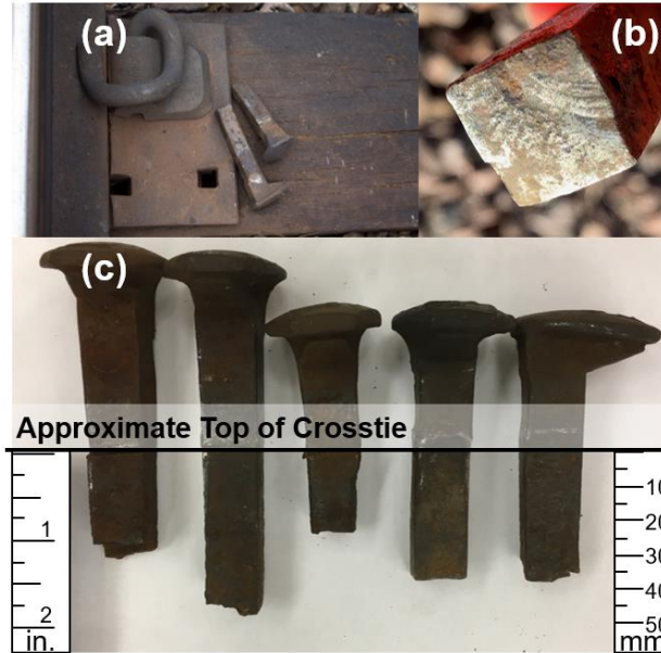
Figure 3.1: (a) A premium fastening system with two broken spikes. (b) Example fracture surface of a broken spike. (c) Examples of broken spikes with varying depths of failure
