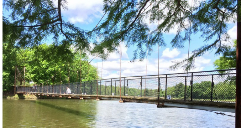
Figure 7.6 Suspension bridge in Lake of the Woods, Mahomet, IL.
