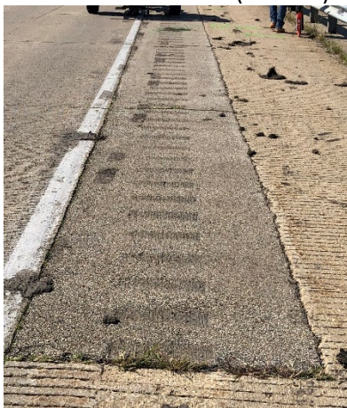
e) HMA partial depth repair along shoulder (901+65 to 904+00)
