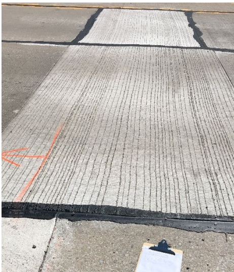
e) Full-depth repairs (12+25 WB)
