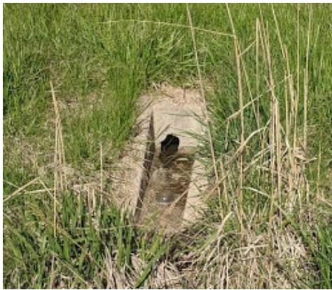
c) Clear drain outlet (26+000 NB)
