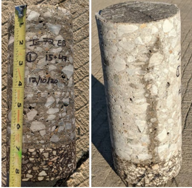
Outer wheel path (approach joint): Over longitudinal crack
