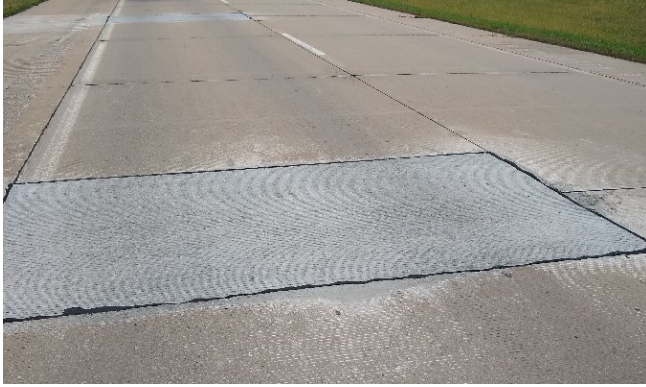
a) New FDR performing well in DL; corner distress in PL along leave joint adjacent to repair (28+660 SB)
