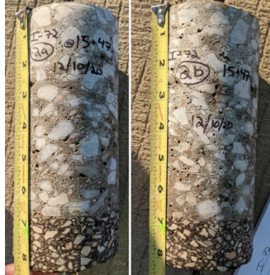
Outer wheel path (approach joint): NOT over longitudinal crack
