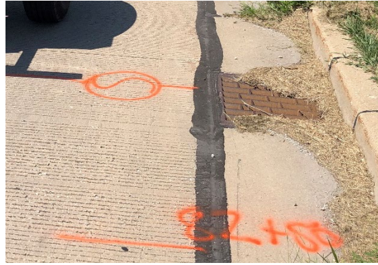
b) Avoided testing over drain locations
