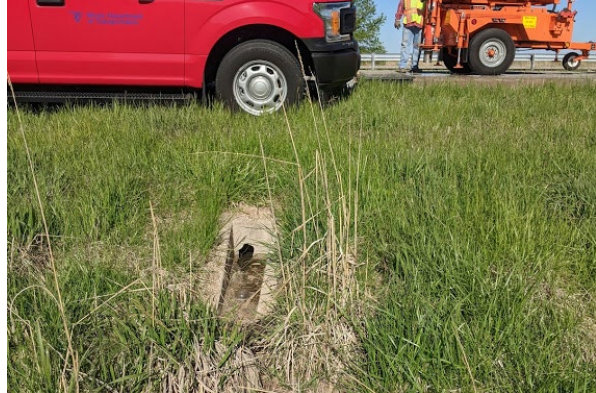
b) NB 26+000 Drain outlet near leave joint
