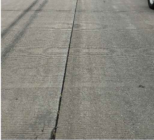
a) Wide longitudinal joint between PL/DL (Section EB-1)
