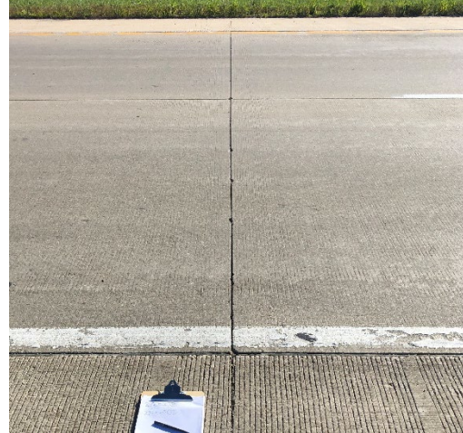
b) Transverse and Longitudinal joints performing well (276+20)
