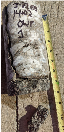
A. 14+02 EB OWP longitudinal crack on leave; stripping on leave only
