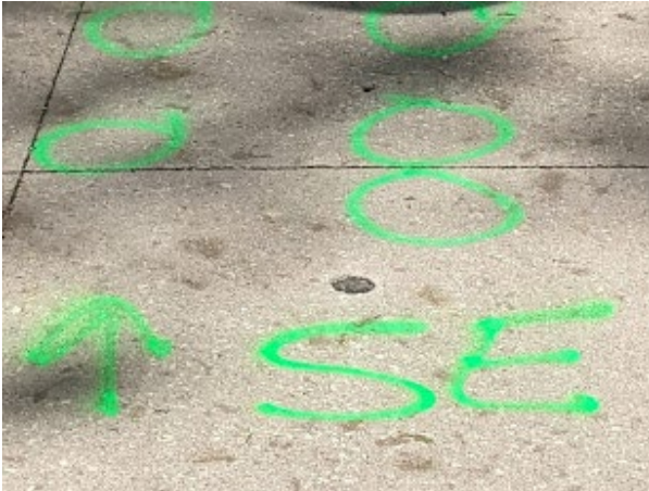
b) Fiber clumping and surface scaling in southeast bay
