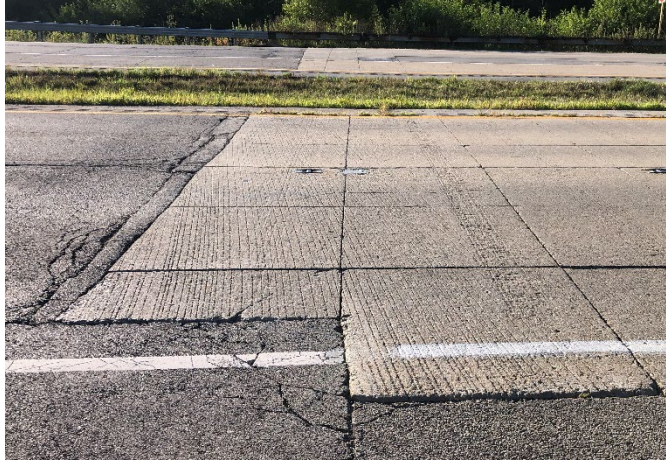
Figure 233. Photo. Start of IL 53 (60N05) SB (assigned stationing of 00+00).
