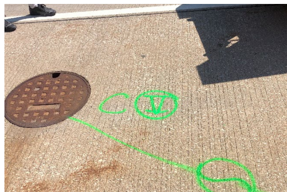
f) Maintenance hole along shoulder (99+65 SB)
