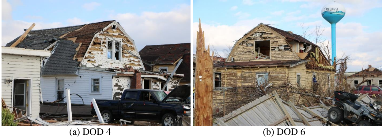
Figure 2.2. Image of residential buildings with DOD rating after the tornado in Naplate, IL: (a) DOD 4 and (b) DOD 6.
