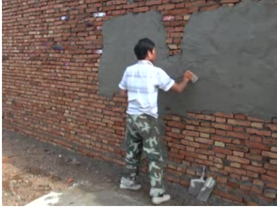
(a) Applying plaster with both arms on or below shoulder level
