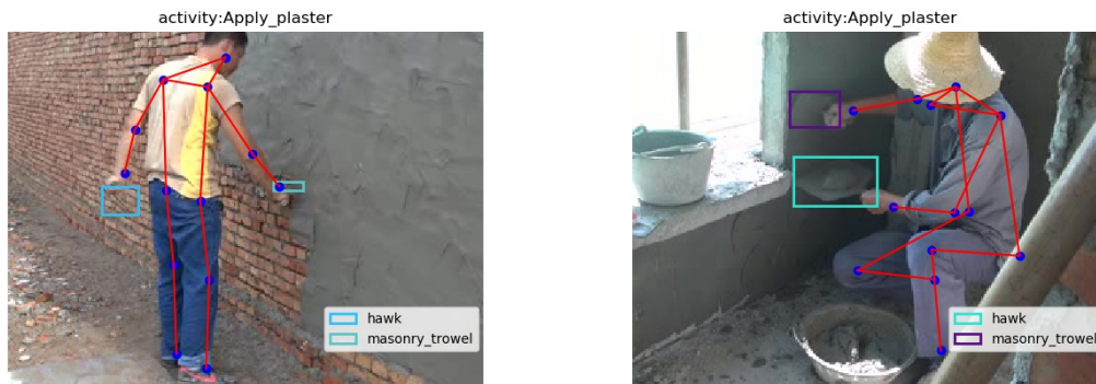
Figure 4.8: Annotation examples of plastering task. Each frame is annotated with an activity label, a set of body keypoints connected by line segments, and a set of object annotations on PPE and tools. Image from dataset introduced in Yang et al. (2016) [53].
