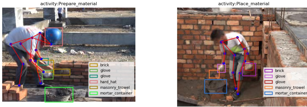
Figure 4.7: Annotation examples of bricklaying task. Each frame is annotated with an activity label, a set of body keypoints connected by line segments, and a set of object annotations on PPE and tools. Image from dataset introduced in Yang et al. (2016) [53].
