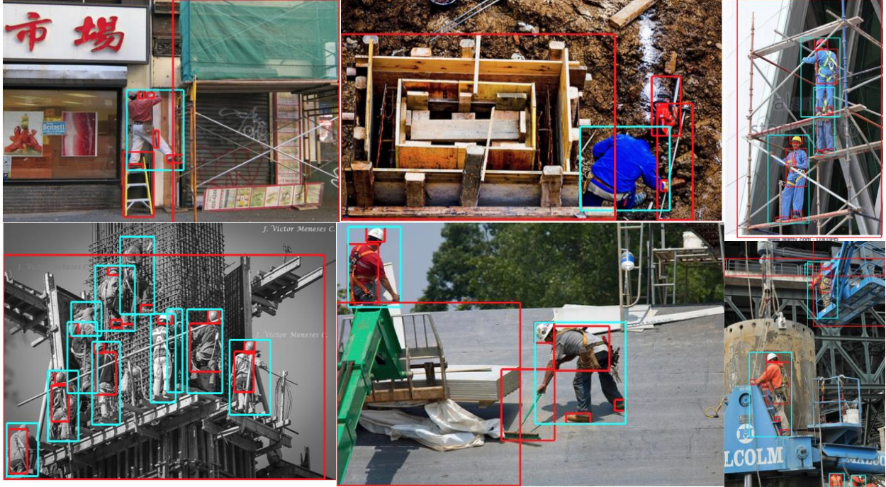
Figure 2.3: Bounding box examples of construction resource instances. Each blue box contains a single worker; red boxes contain instances of other object categories that a worker might interact with.
