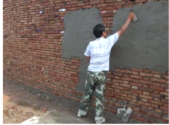
(b) Applying plaster with one arm above shoulder level
