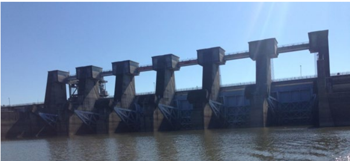
Figure 2.16. Series of Tainter gates at the dam portion of a lock and dam.
