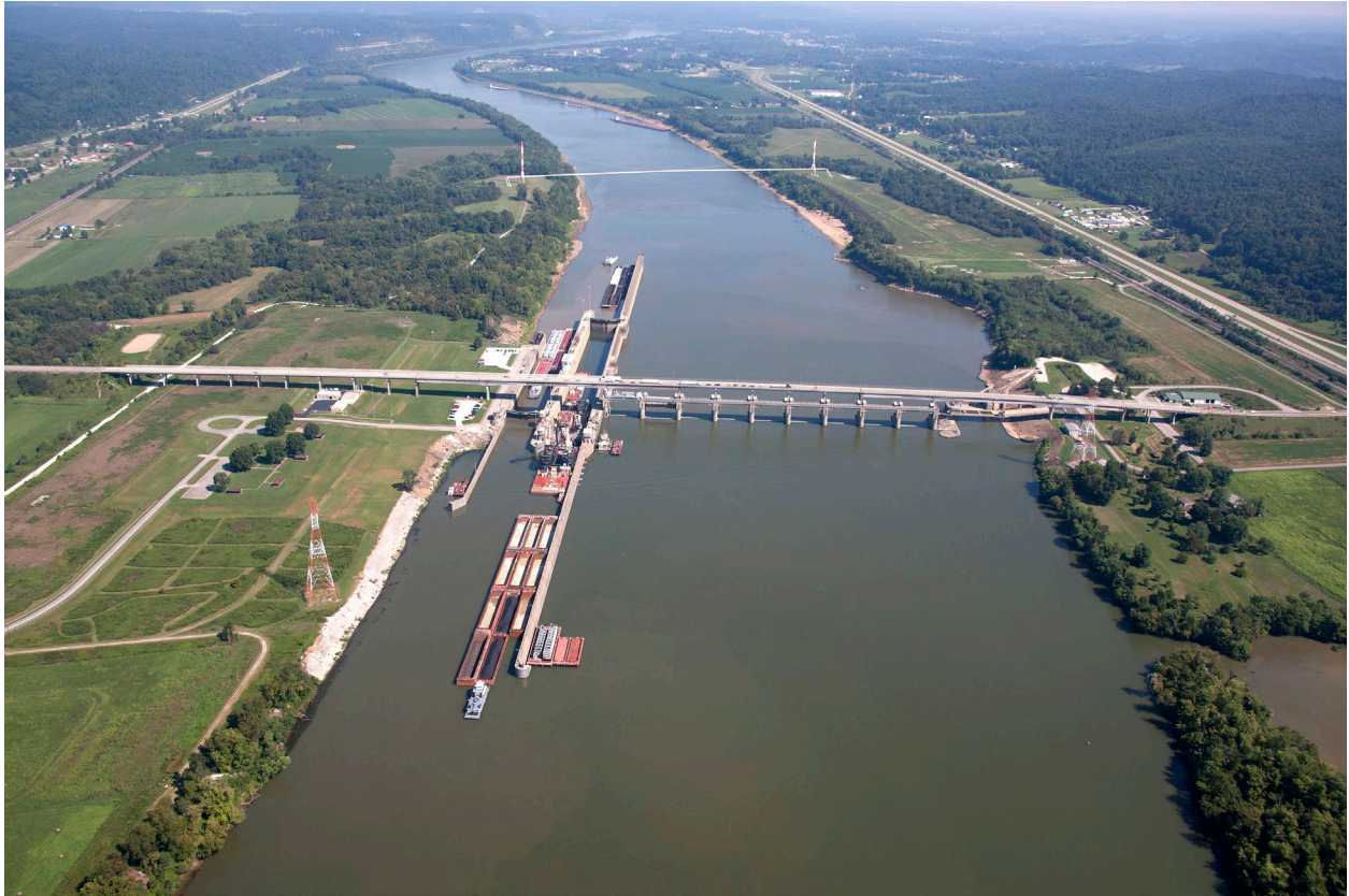
Figure 1.3. The Greenup Lock and Dam site on the Ohio River (U.S. Army Corps of Engineers n.d.).
