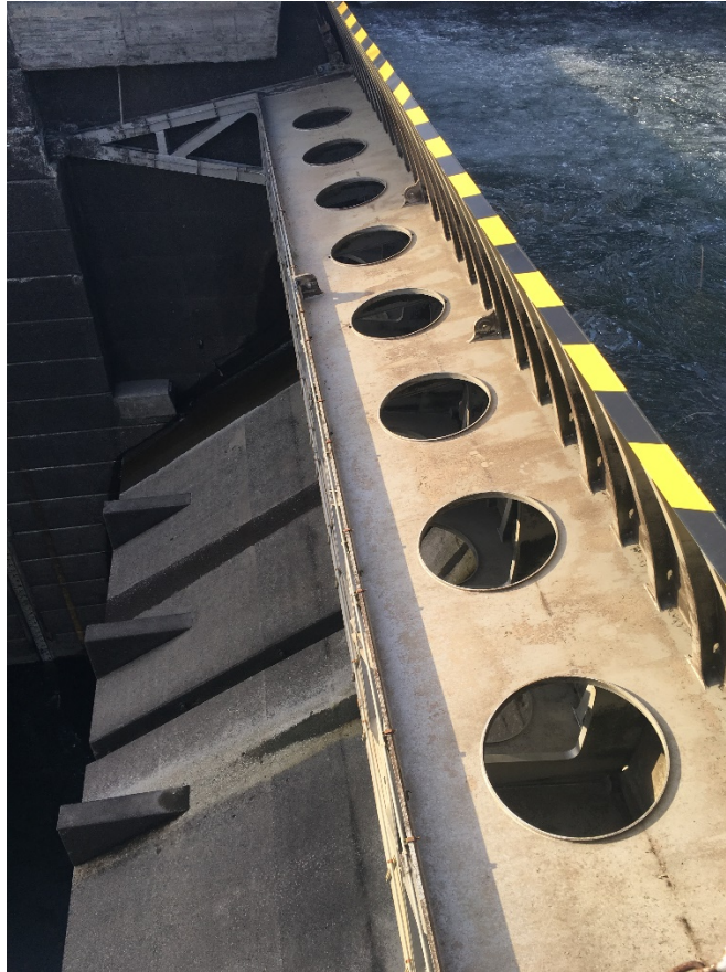
Figure 6.1. Tainter lock gate at The Dalles, closed and acting as the damming surface to the lock chamber.
