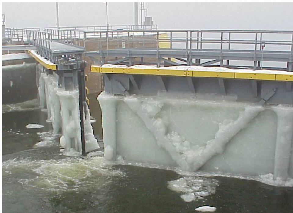
Figure 1.9. Miter gate mostly submerged and encased in ice (Mulherin and Haehnel 2003).
