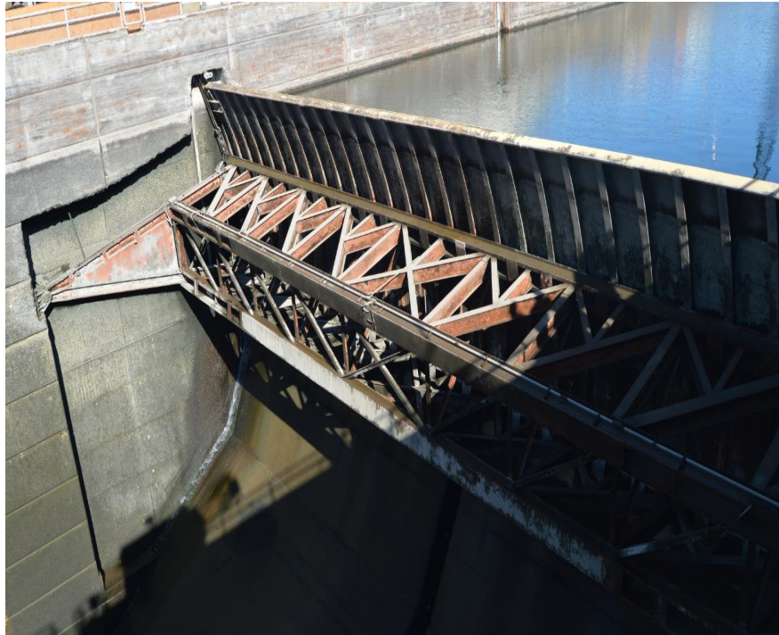
Figure 2.18. The Dalles Tainter gate, closed and acting as the damming surface of the lock chamber.
