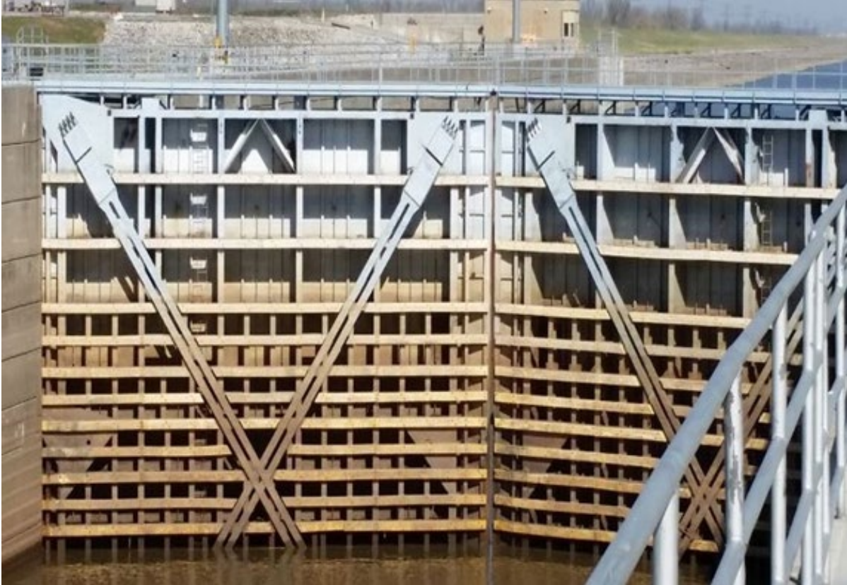
Figure 1.5. Horizontally framed miter gate at Lock 27 on the Mississippi River.
