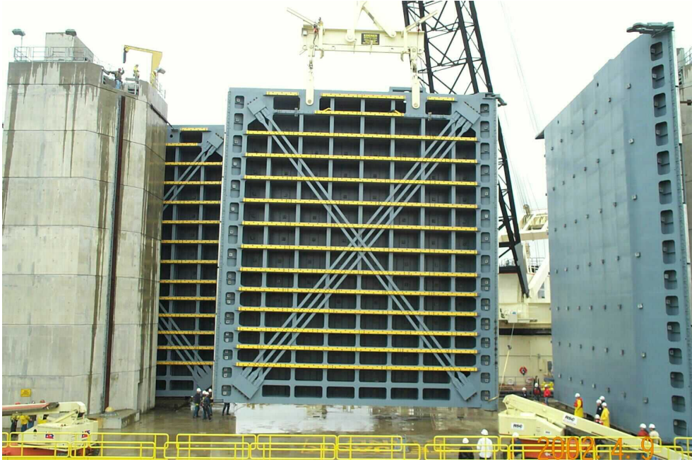
Figure 2.1. Horizontally framed Miter gate being installed in the field.
