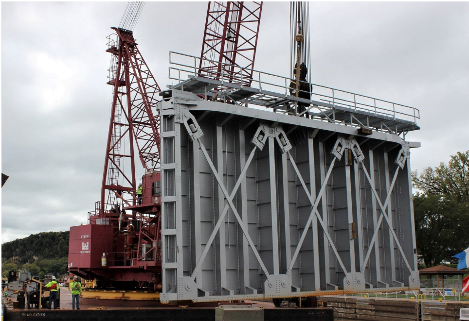
Figure 2.2. Vertically framed miter gate being installed in the field.
