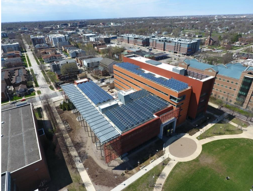
Figure 26: Drone shot of the rooftop solar panels
