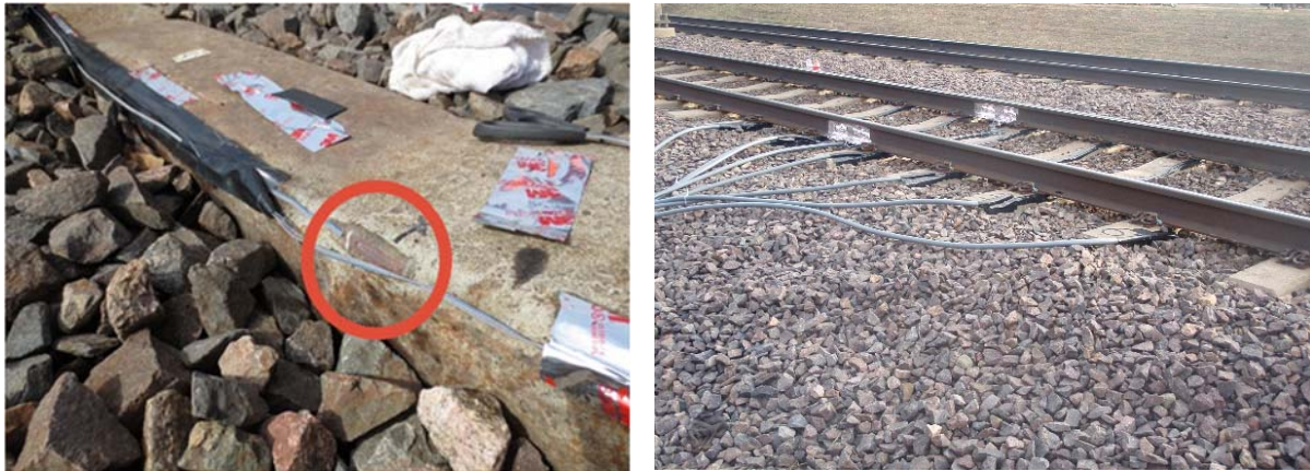
Figure 4.3: Crossties instrumented with concrete surface strain gauges and the completed St. Louis MetroLink light rail field experimentation location.
