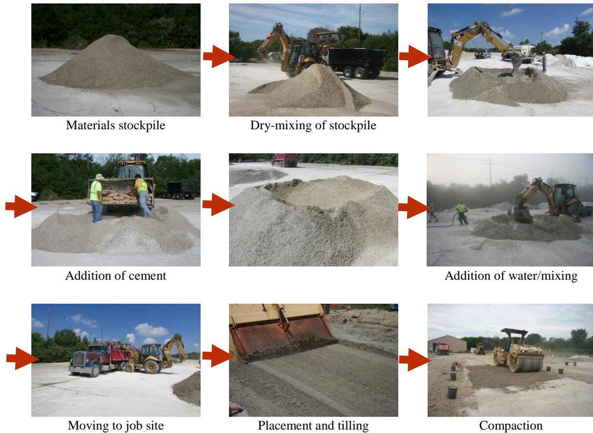
Figure 4.13 Construction steps of chemically stabilized test sections in Cells 2 and 3
