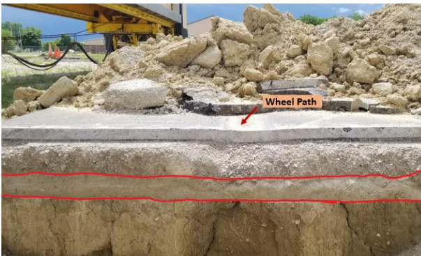
C3S3W – QB2 + Fly Ash Subbase & CA06_R Base
