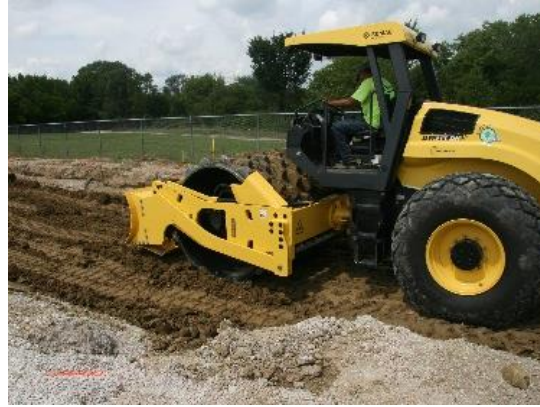
Subgrade compaction
