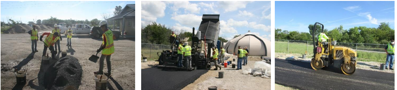
Figure 4.15 Hot mix asphalt sampling and paving
