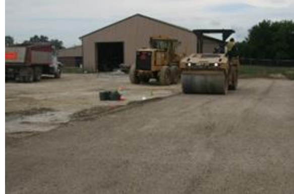
Placement of CA06_R capping layer for Cell 1
