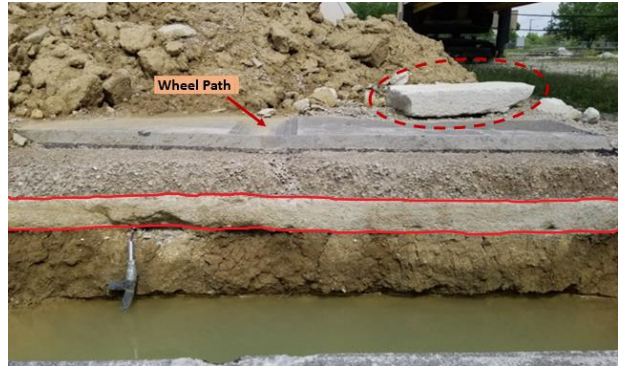
C3S2E – QB2 + Cement Subbase & CA06_R Base
