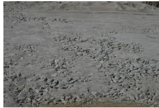
Final compacted surface of C1S1
