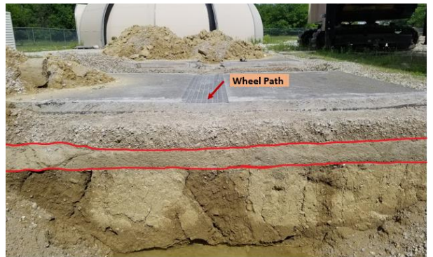
C323E – QB2 + Fly Ash Subbase & CA06_R Base
