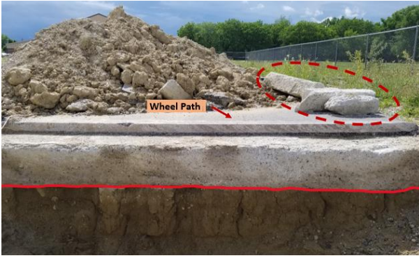
C2S1W – QB2 + FRAP + Cement
