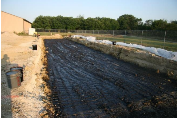
Subgrade surface after application of tack coat
