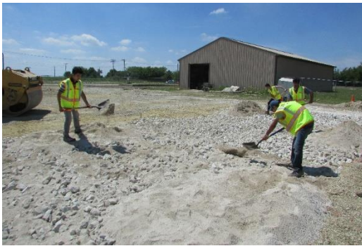
Uniform spreading and incremental placement of QB1 on top of PCR lift
