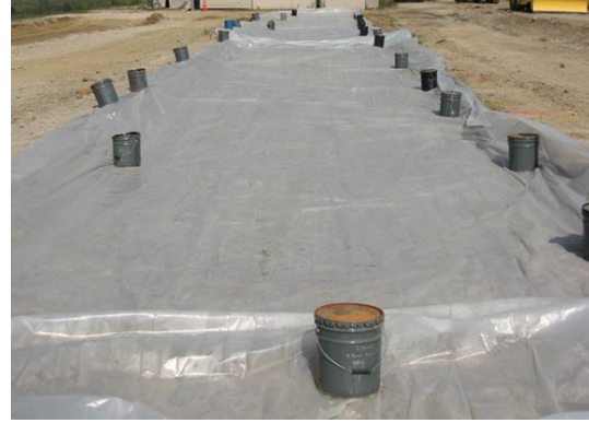
Test Cells covered with plastic sheets
