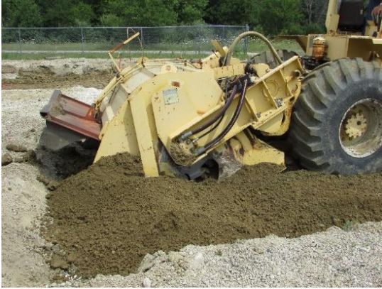
Subgrade soil tilling and mixing
