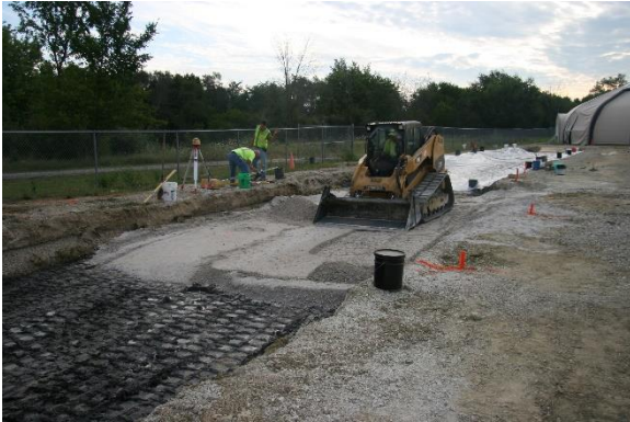
Construction of C1S4 unbound layers
