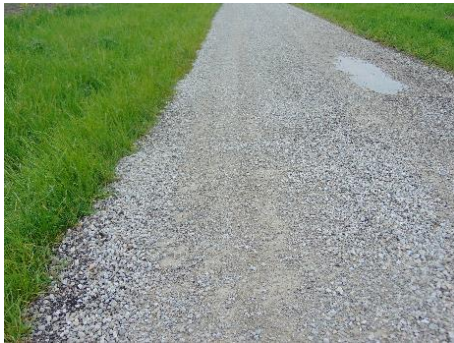
(a) Gravel road
