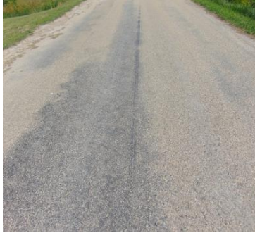
Figure 11. Polished aggregate in seal-coated road.
