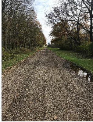
(a) Gravel road
