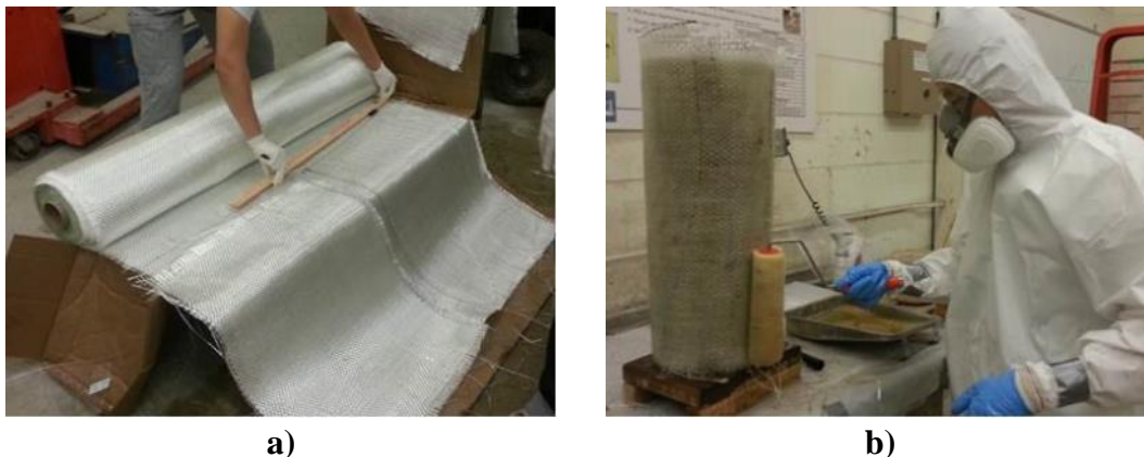
Figure 3.2 FRP wet layup process a) cutting the fabric b) resin application
