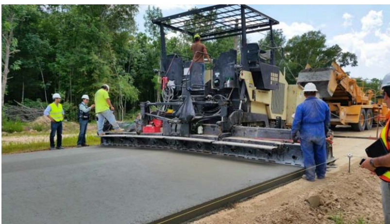
Figure 1. High-density paver placing RCC pavement from Prusinski (2016).
