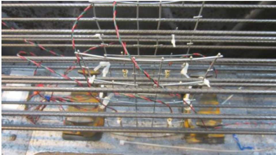
Figure 3.14 Mesh to Hold Embedment Crosstie Strain Gauges Prior to Concrete Being Poured
