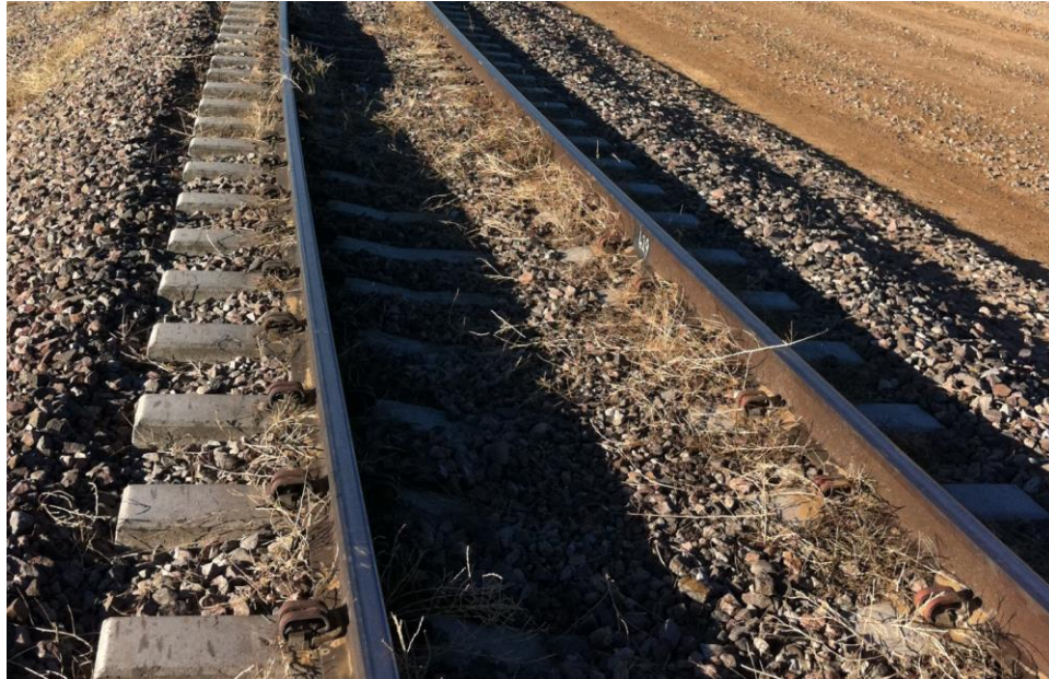
Figure 1.1 Use of Crossties in Track System
